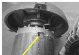
Drilled hole in the end ring
